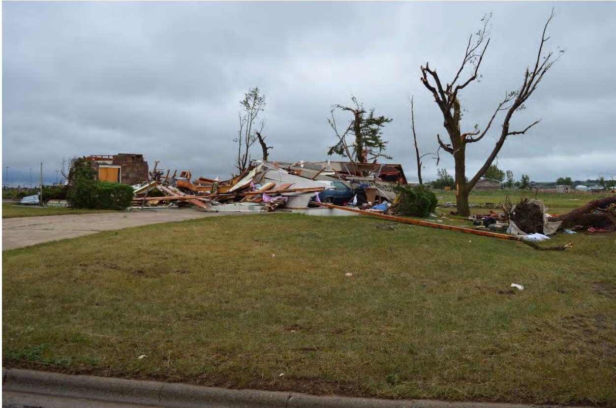
Figure 5: Home destroyed from the 2016 Tornado in Baker
